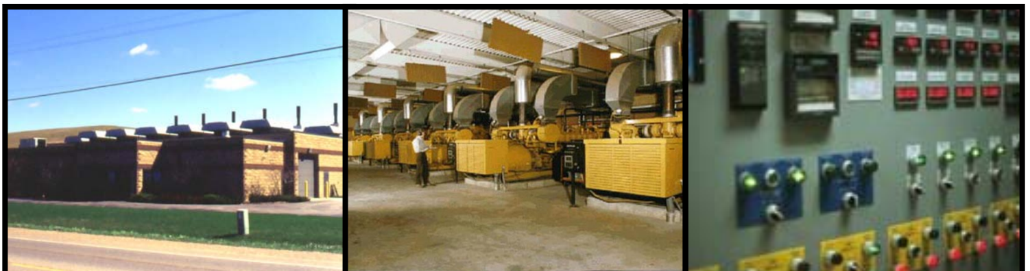
Ottawa Generating Station Exterior
